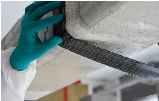
Apply the folded S&P C-Sheets according to the instructions for single layer S&P C-Sheets (see Application Instructions S&P C-Sheet).
