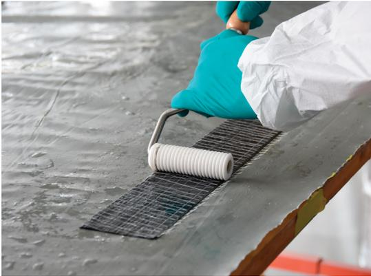
Following the folding, work more epoxy resin into the S&P C-Sheet using a rubber spatula (squeeze) and a teflon roller. Again, only apply the resin **in the direction of the fibres (longitudinal)**.
