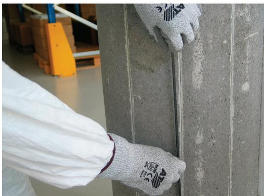
Insert the S&P C-Laminates into the slots.
