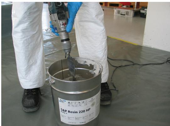
Mix S&P Resin 220 HP on low-speed, max. 400 RPM.
