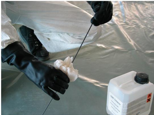
Clean and degrease laminates on both sides with a clean towel and S&P Cleaner.
