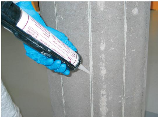
Fill the slots with S&P Resin 220 HP.
