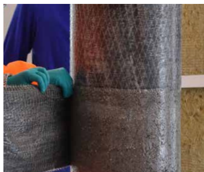
Axial column reinforcement with S&P C-Sheet 240
