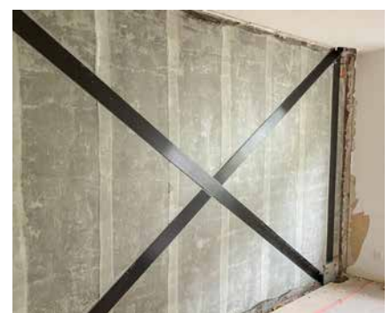
Seismic reinforcement with S&P G-Sheet and S&P C-Laminate
