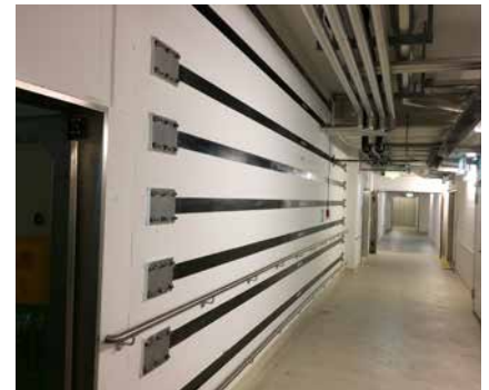
Shear reinforcement with pre-stressed S&P C-Laminate
