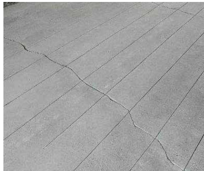
Flexural reinforcement with near surface mounted (NSM) S&P C-Laminate
