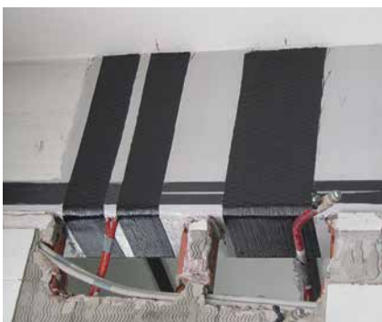
Shear reinforcement with S&P C-Sheet 640
