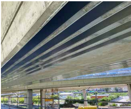
Flexural reinforcement with externally bonded S&P C-Laminate
