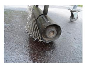
Roll onto the S&P asphalt reinforcement with the roller – the plastic film should be face-down onto the bonding agent.
