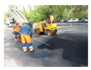
S&P recommends spreading asphalt over the locally unrolled reinforcement.
