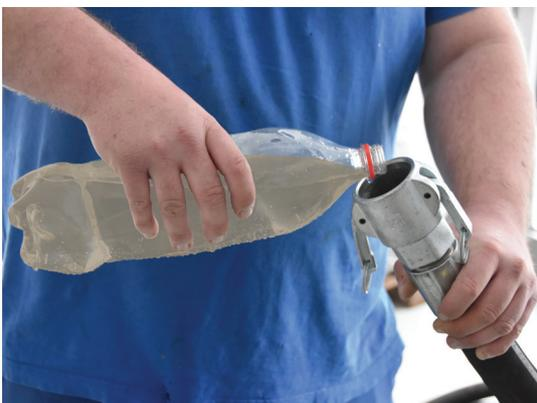
Before starting the material conveying, a lubricating mixture must be added to the material hoses! This can be a cement slurry, but we recommend using fish paste.
