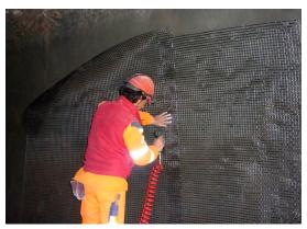
After about 3~4 hours, the S&P carbon fibre reinforcement mesh can be fixed to the substrate with staples (special Inox-shape) and a pneumatic staple gun. The staple gun is operated with a small air compressor.
