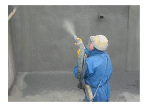
Apply the first layer of S&P ARMO-crete® d on the clean, slightly damp and dust-free substrate.
