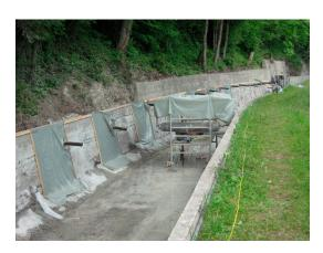
After the application, the shotcrete mortar should to be protected against draying out (sun and wind exposure), and must be kept moist for up to 7 days.
