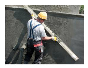
Treatment of surface according to the requirements. The carbon fibre reinforcement mesh must be covered in about 1 cm, up to 2 cm.
