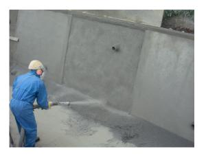
The substrate should be cleaned thoroughly with water pressure of about 150 bar before applying the second layer of shotcrete mortar.
