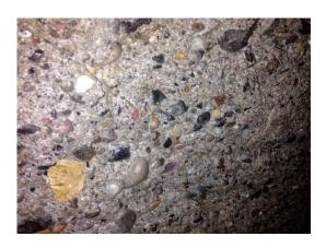
On the previous day, water the bearing substrate to full capillary saturation. The roughness should be 3-5 mm.
