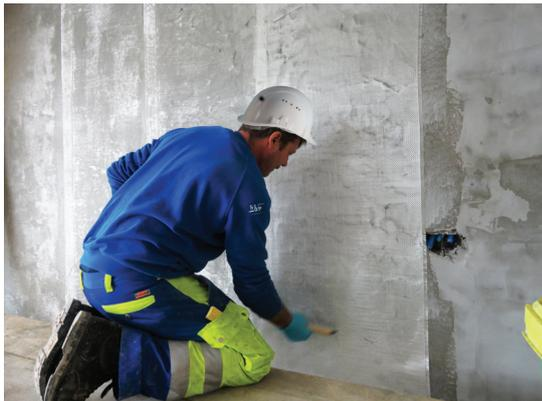
Always roll in the direction of the fibre, and do so until all fibres are moistened and there are no air pockets left in the sheet.
