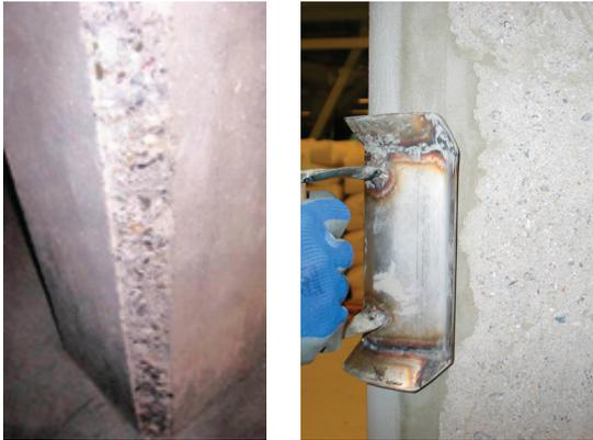
Round off corners and edges within a radius of 25 mm (chamfer or re-profile).
