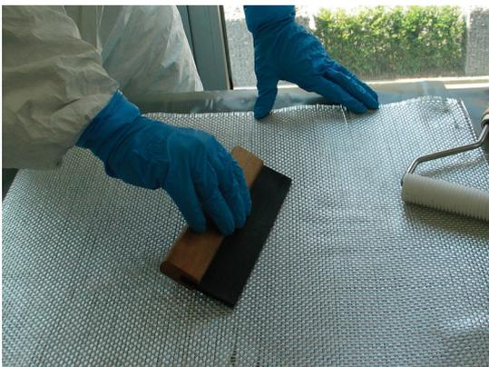
Pre-impregnate the S&P G-Sheet E/AR with S&P Resicem HP or S&P Resin 55 HP.
