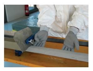
Apply the glue onto the clean side of the laminate in a dome shape.
