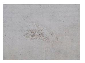
Remove bad concrete (honeycomb), uneven surfaces, loose material, wood pieces, insulation material etc.
