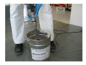
Mix S&P Resin 220 HP at low speed, maximum 400 RPM.
