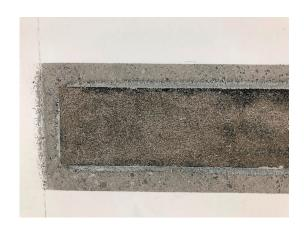
For a subsequent application of plaster, the laminates must be covered in quartz sand.
