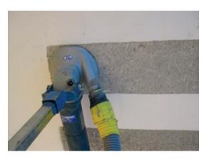
Sand blast, shut blast, or grind the substrate with a cup wheel. Not using a chisel!
