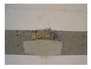
Reprofile using epoxy-based S&P Resin 230 HP levelling mortar
