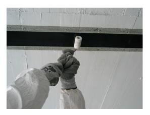
Press the laminate onto the substrate using a Teflon roller from the centre out to each extremity.
