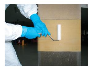
The roller must only be rolled in the direction of the fibre until all fibres are moistened and there are no air pockets left in the sheet.
