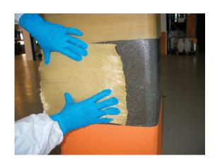
Fix the pre-impregnated S&P A-Sheet 120 onto the substrate.
