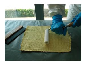
Pre-impregnate the S&P A-Sheet with S&P Resicem HP or S&P Resin 55 HP.
