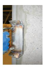
Round off corners and edges within a radius of 25 mm (chamfer or re-profile).
