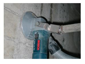
Sand blast, shut blast, or grind the substrate using a cup wheel. Not using a chisel!
