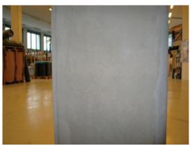
Re-profile using S&P Tecnogrout-K or S&P Resin 230 HP.
