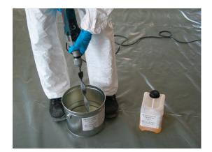
Mix the adhesive at a low speed, max. 400 RPM.
