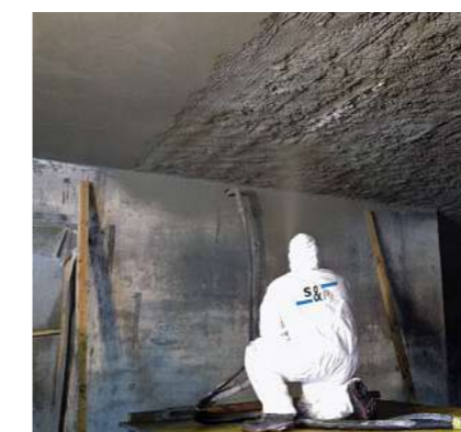
4 Building construction (seismic retrofit, reinforcement of columns)
