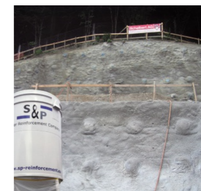
5 Civil engineering (ensuring the safety of excavations, retaining walls)
