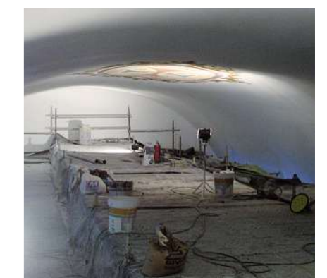
6 Historical buildings (reinforcement of masonry)
