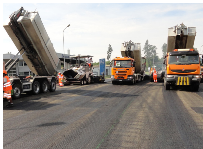
5 Same day asphalt overlay installation
