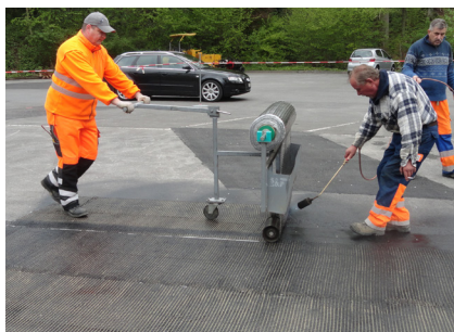
4 Manual application of S&P reinforcement grid for local reinforcement
