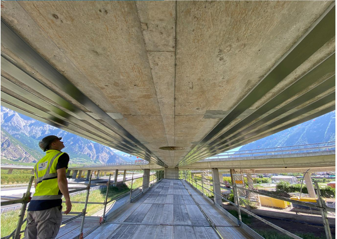
▲ Span of 26m, reinforced with various S&P C-Laminate.
