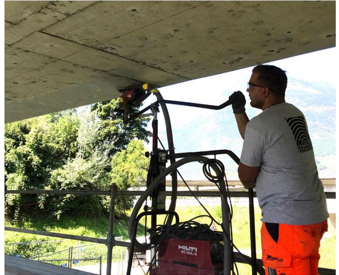
▲ The preparation included marking and grinding the concrete substrate with an extended grinder
