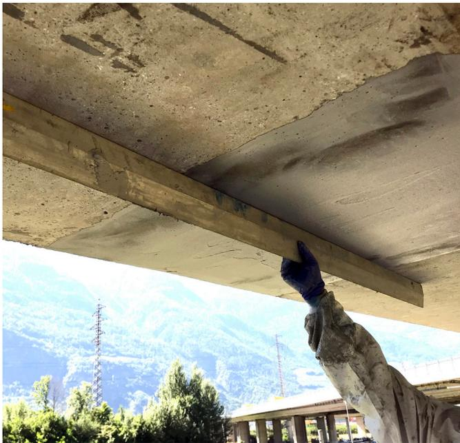
▲ Checking the evenness of the substrate after reprofiling slight irregularities with S&P Resin 220 HP
