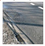
Substantial cracking could already be seen on areas of the road where no S&P asphalt reinforcement grids were installed.
