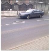
Finally after 8 years, the first signs of damage began to appear and the thinness of the asphalt layer on top is clearly visible.
