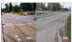
In the areas where S&P asphalt reinforcement grids were installed, no damage was observed - complete contrast to sections of road with no grid.
