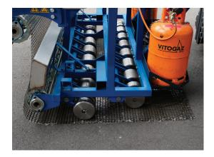
Lower the unrolling machine to the ground, ignite the burner, close the wind protection and drive forwards.
