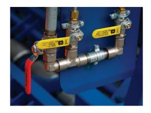
Open the gas canister, pull the red gas lever downwards.
