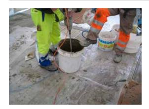
Mix the S&P ARMO-crete® w bag of 25 kg with 3.6~3.8 liter of water - depending on the consistency of the shotcrete mortar. Mix with a mechanical mixer for at least 3 minutes until the mixture is homogeneous. The mixture should rest 1 minute, then be re-mixed for another 10 seconds before application.
