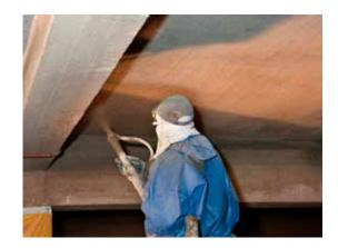
Apply the second layer of S&P ARMO-crete<sup>®</sup> w onto the uncured first layer of mortar (wet on wet). Once the setting process has started, the mortar can be troweled up and grinded to the desired thickness.
