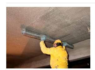
Incorporate the S&P ARMO-mesh® into the fresh S&P ARMO-crete® w. This is done by pressing the S&P ARMO-mesh® into the mortar using a trowel. Ensure that the fibers of the reinforcement are stretched out as much as possible.
