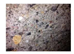
On the day prior to the application, water the bearing substrate to full capillary saturation. The roughness should be 3-5 mm.
