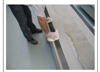
Using S&P Cleaner, clean and remove any grease on the glue-applying side of S&P laminates and end anchors.
