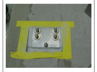
Press the bottom anchor plate into the recess and lightly tighten all the bolts (M12)
