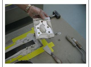
Likewise, coat the top anchor plate in S&P Resin 220.
