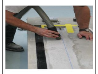
In the area where the laminate will be installed, the bearing substrate must be cleaned thoroughly using a vacuuming hose.
