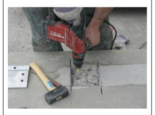
Drill and insert the dowel (1 x M12). The thread must protrude by at least 40 mm.
