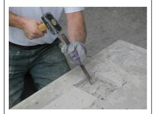
Remove the concrete in the recess area.
