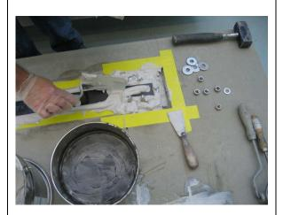
Stick the laminate onto the substrate correctly and professionally. Coat the anchoring ends with glue.
