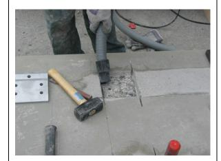
Remove all dust on the bearing substrate completely by using a vacuum hose.
