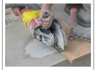
Start to cut the front side (adjacent to the laminate) of the recess with a diamond blade.
