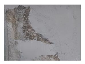
Remove damaged concrete (honeycomb), masonry, loose material, wood pieces, insulation material etc.
