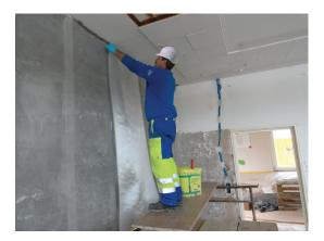
Fix the pre-impregnated S&P G-Sheet E/AR onto the substrate.
