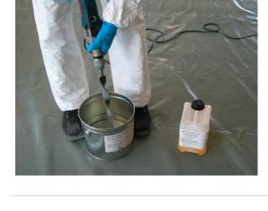
Mix the adhesive at a low speed, max. 400 RPM.
