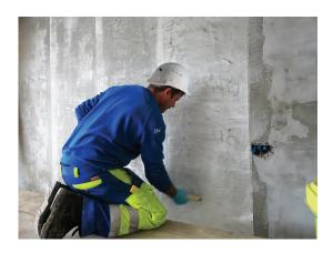
Always roll in the direction of the fibre, and do so until all fibres are moistened and there are no air pockets left in the sheet.
