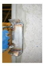
Round off corners and edges within a radius of 25 mm (chamfer or re-profile).
