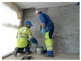
Apply S&P Resicem HP (improves vapour exchanges) or S&P Resin 55 HP (vapour proof) onto the substrate.
