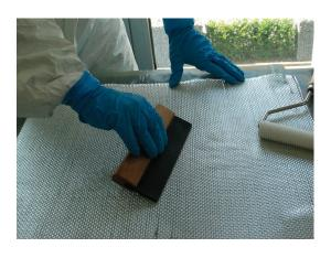
Pre-impregnate the S&P G-Sheet E/AR with S&P Resicem HP or S&P Resin 55 HP.
