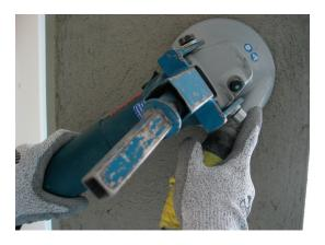
Sand blast, shot blast or grind using a diamond cup wheel.
