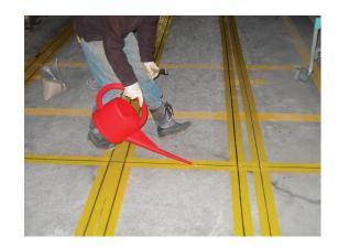
When applying on horizontal building components, the slots can also be filled with S&P Resin 55 HP.
