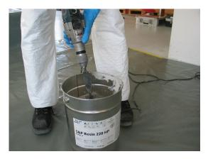
Mix S&P Resin 220 HP on low-speed, max. 400 RPM.
