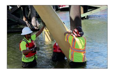
Install a bead of FX-763CTG into the locking groove of the jacket and place FX-70<sup>®</sup> jacket around the pile to be repaired.
