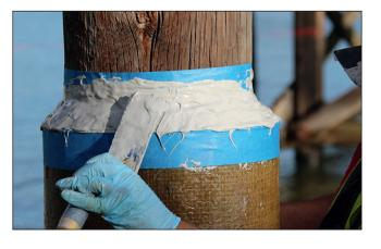
Install FX-763 Trowel Grade Epoxy at the head of the jacket and finish to a 45° tapered bevel, creating a water and chemical resistant barrier to the repair system.
