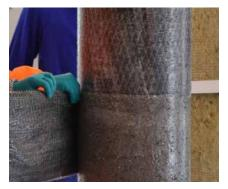
Axial column reinforcement with S&P C-Sheet 240
