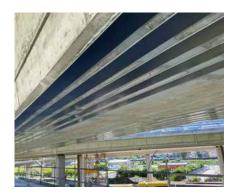
Flexural reinforcement with externally bonded S&P C-Laminate
