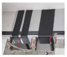
Shear reinforcement with S&P C-Sheet 640
