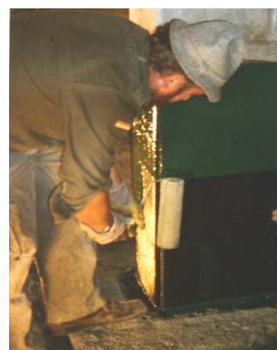
Fig. 4: Impregnation of the sheet with S&P Resicem (vapour permeable)
