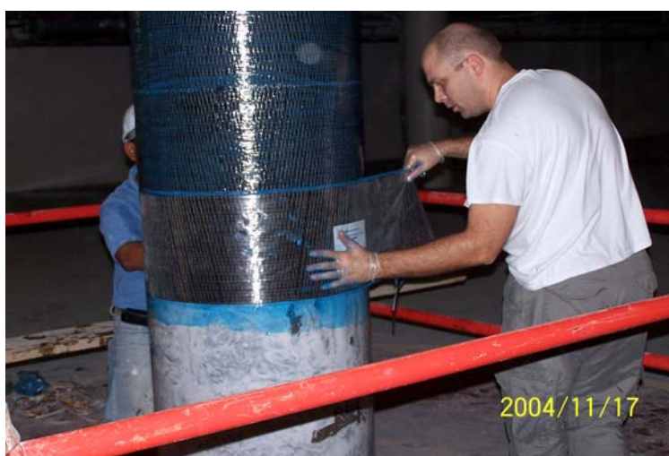
Fig. 4: Impregnation of the sheet with S&P Resicem (vapour permeable)
