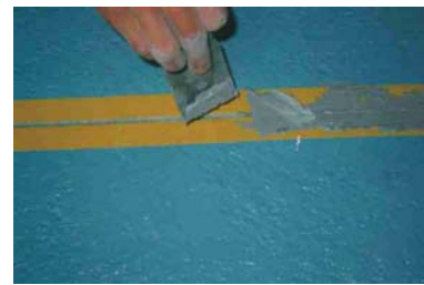
Fig. 2: Bonding with slots
