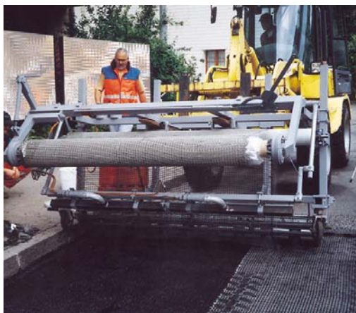
Image 9: Application of S&P Carbophalt G
